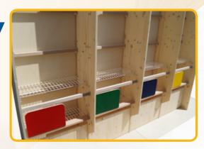
Now the wire meshes are inserted. The folds must point downwards. Tip: Insert the wire meshes before the coloured rotatable panels are fitted.
