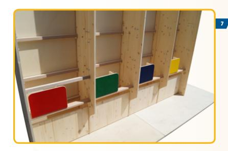
Fit all the rotatable panels marked with the number 1 into the bottom section rows.
