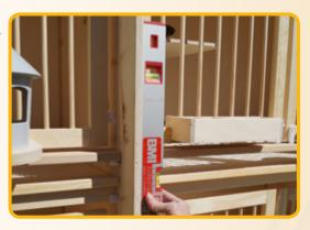
The sectioned box must now be aligned with the spirit level and securely screwed to the rear wall.
