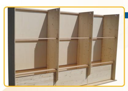
Press the beech wood perch bars onto the metal bolts on the upright side walls. In doing so, the short clearance of the two slots on the perch bars must point to the front.
