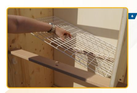
Now the wire meshes are fitted. The folds must point downwards.
